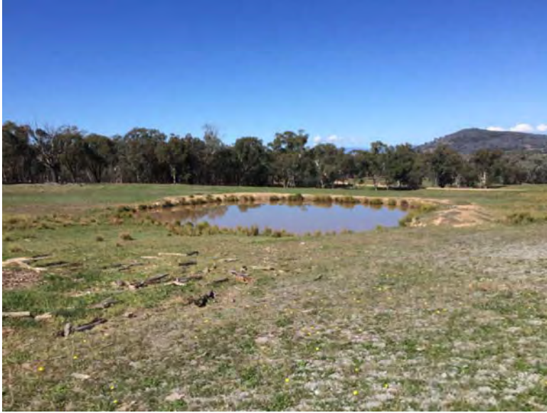
Figure 15 Detention dam located to the south of Pit 1.
