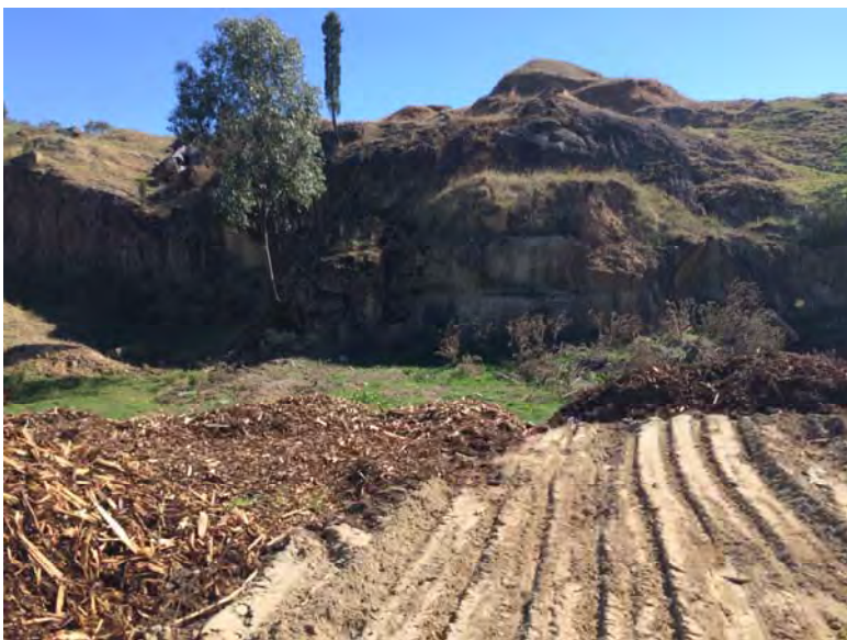
Figure 14 Example of site rehabilitation works occurring within Pit 1
