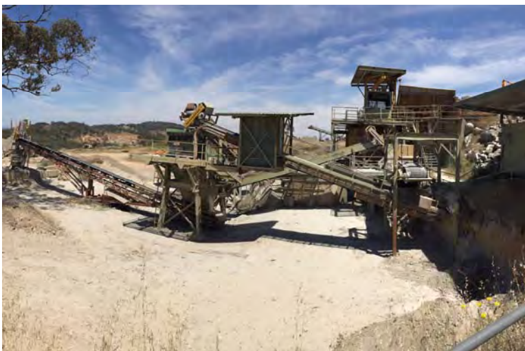
Figure 20 Crushing and screening plant contained within Pit 3.
