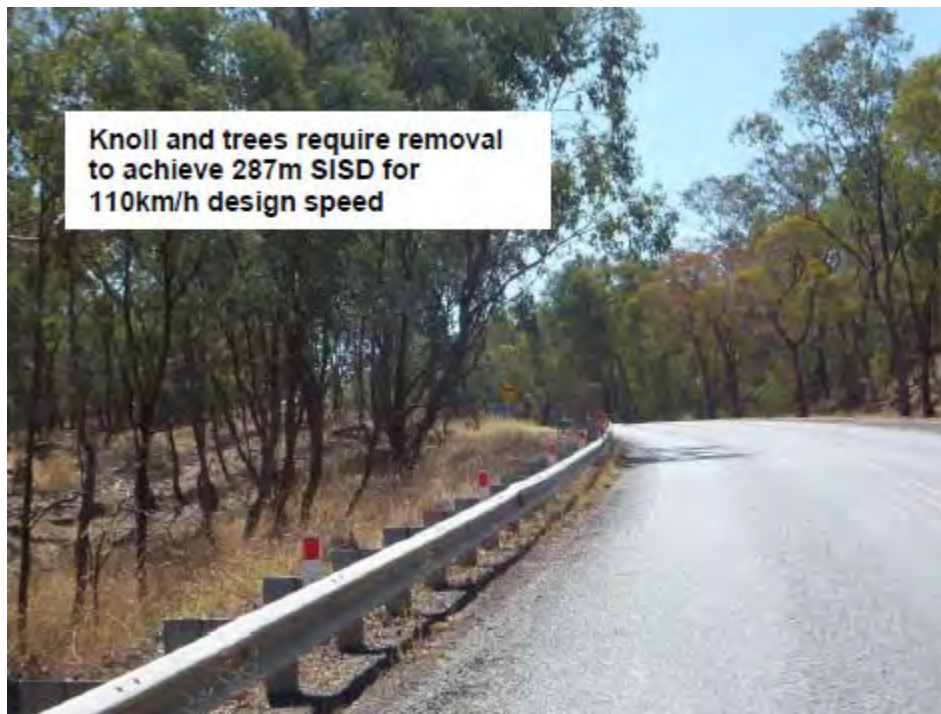
Figure 46: Gerogery Road north bound at 287m from Winchester Lane (Source: Traffic Impact Assessment, Rockwood Quarry Winchester Lane, Peter Meredith Consulting, 2018)
