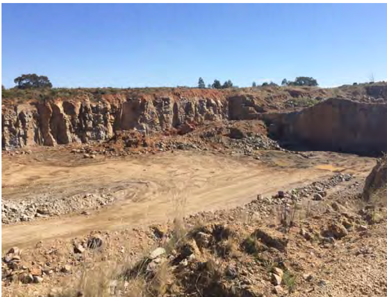
Figure 17 Pit 3 extraction area looking west.
